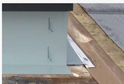
Plug-in plinth before gluing-in
