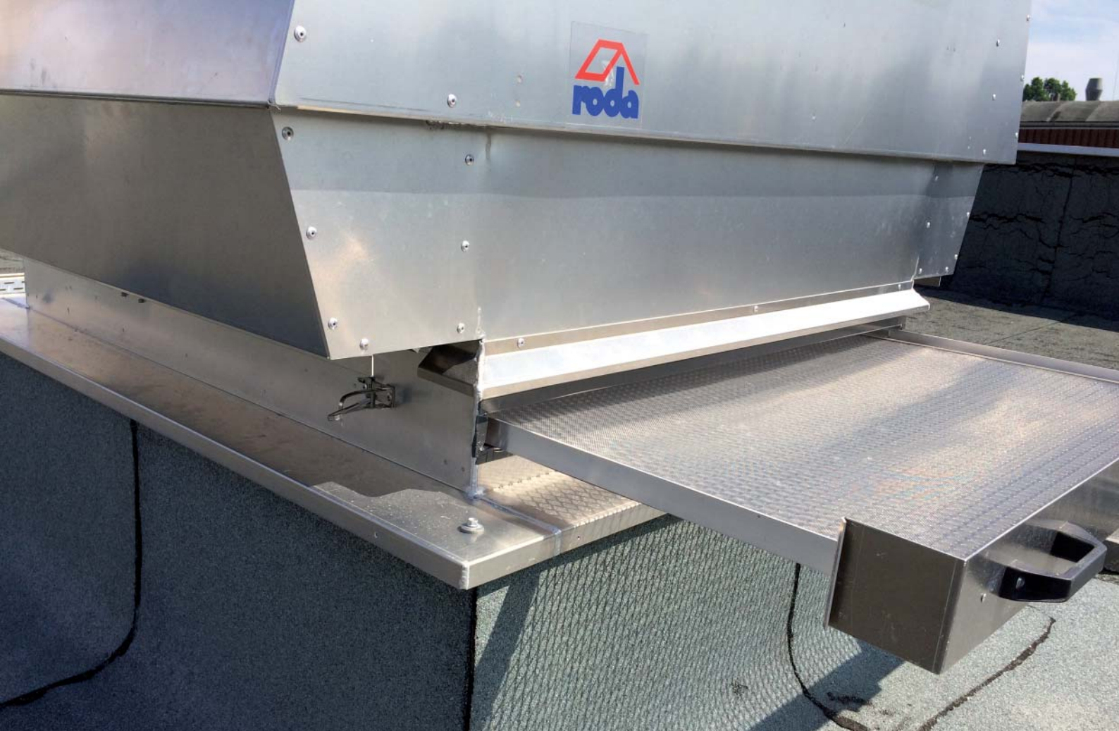
In closed position the drawer is fixed by tension latches.
