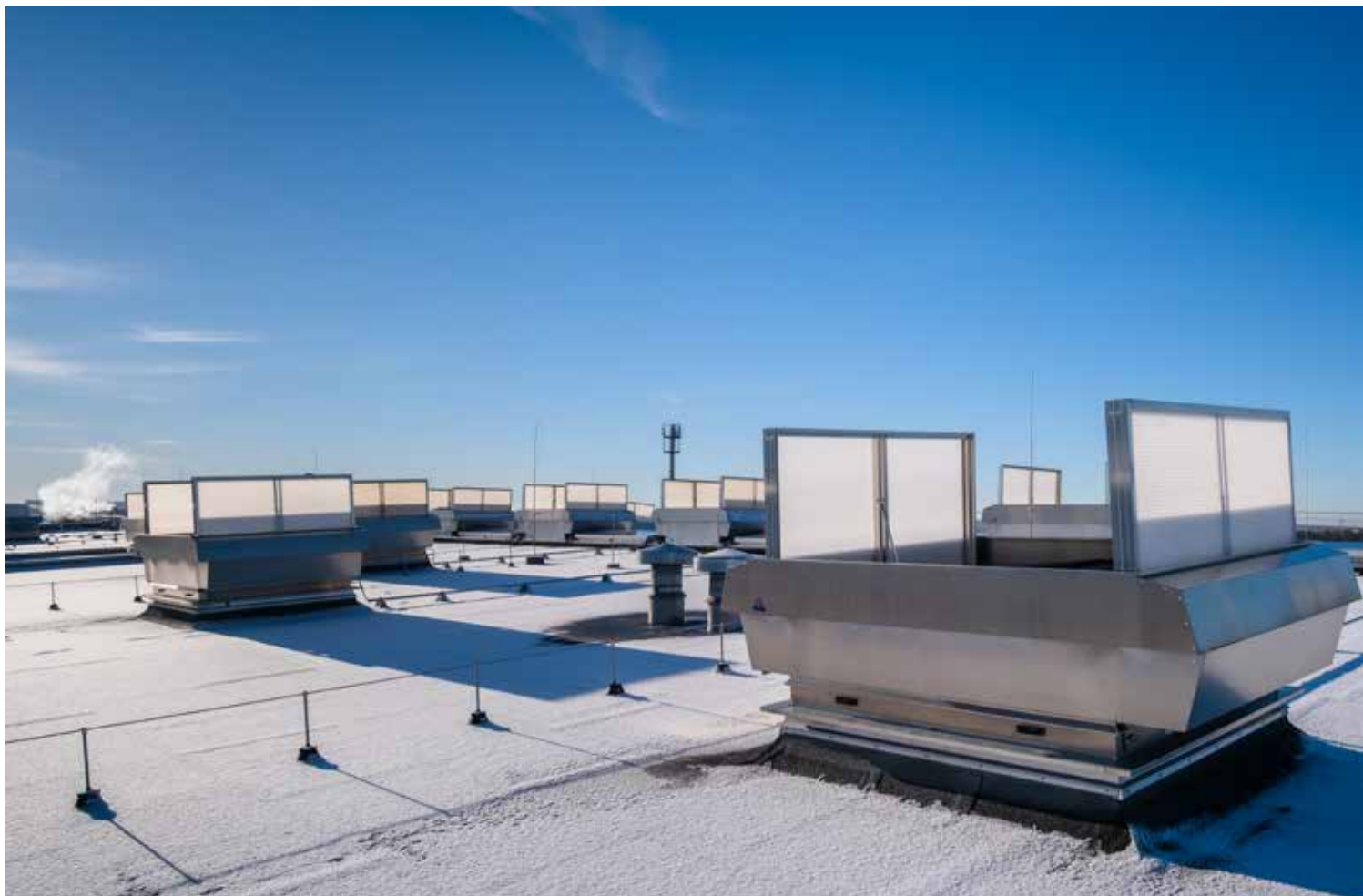
MEGAPHÖNIX in ventilation position 90° for maximum natural air exchange
