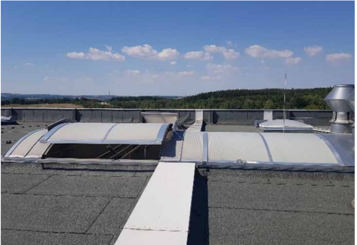
Before: Continuous rooflights, rooflights and ventilation flaps
