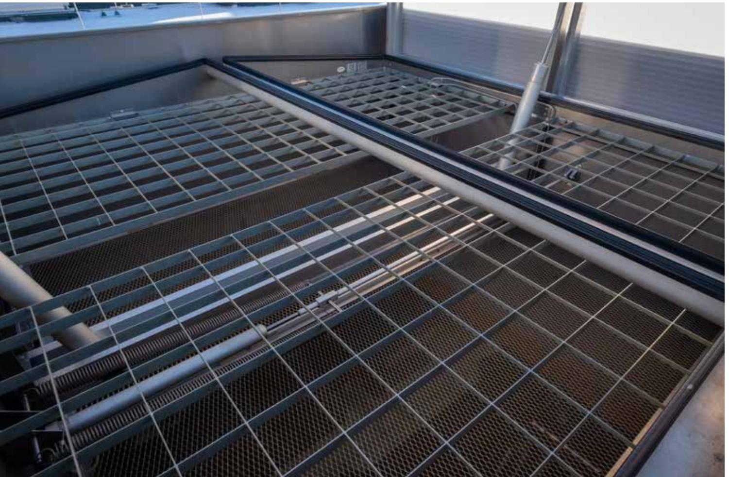
Fall-through grilles for more safety on the roof during cleaning and maintenance work and insect screens for hygiene protection
