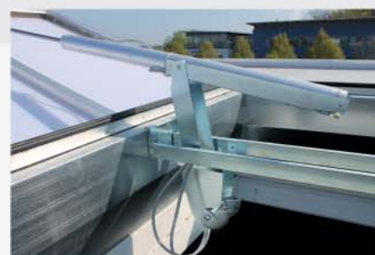
Pneumatic drive with one cylinder
