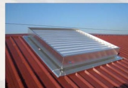
Connected to a trapezoidal gable roof
