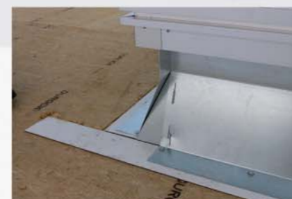
Plug-in plinth before gluing-in
