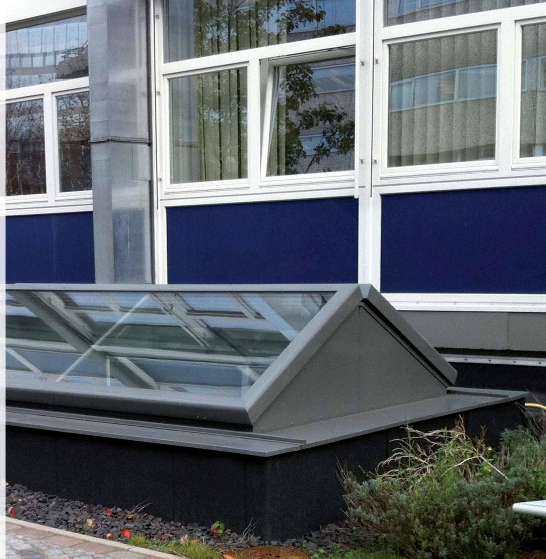
Large picture: FIREFIGHTER DELTA as a natural and heat extractor for the ground floor
