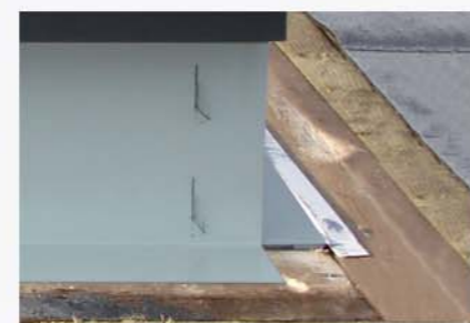
Plug-in plinth before gluing-in
