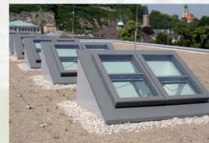
Mounted on a sloped plinth
