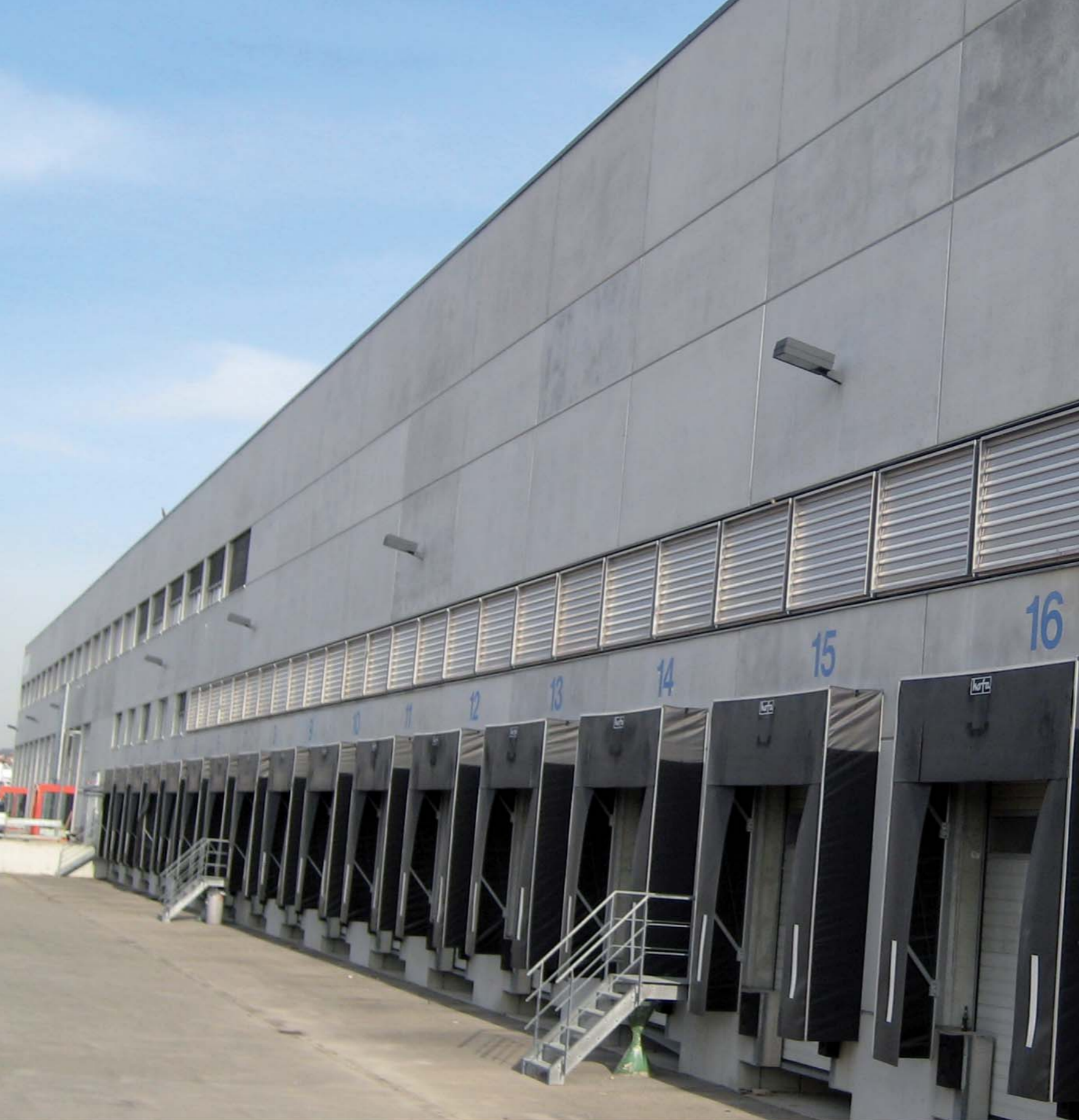
Large picture: SMOKEJET as an air supply unit in the wall
