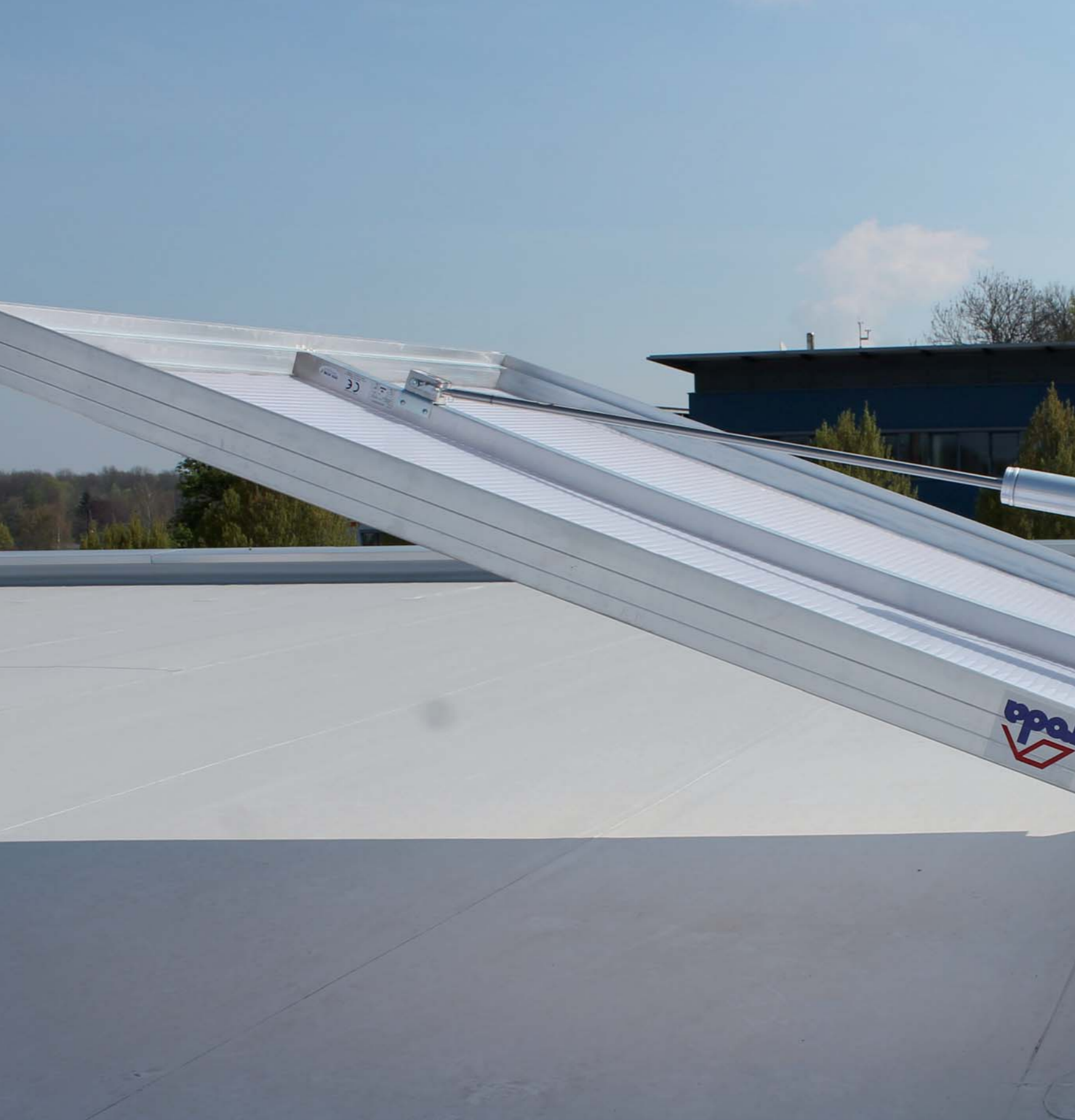
Picture: VenturiSmoke VS1 on a food company's roof, opened for daily ventilation
